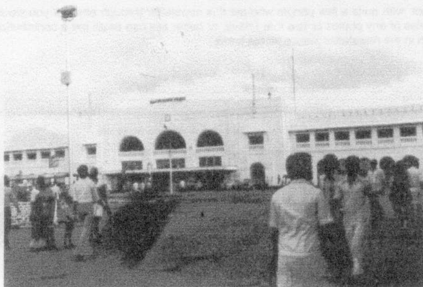
A recent photograph of the modern railway station at Tiruchirappalli
