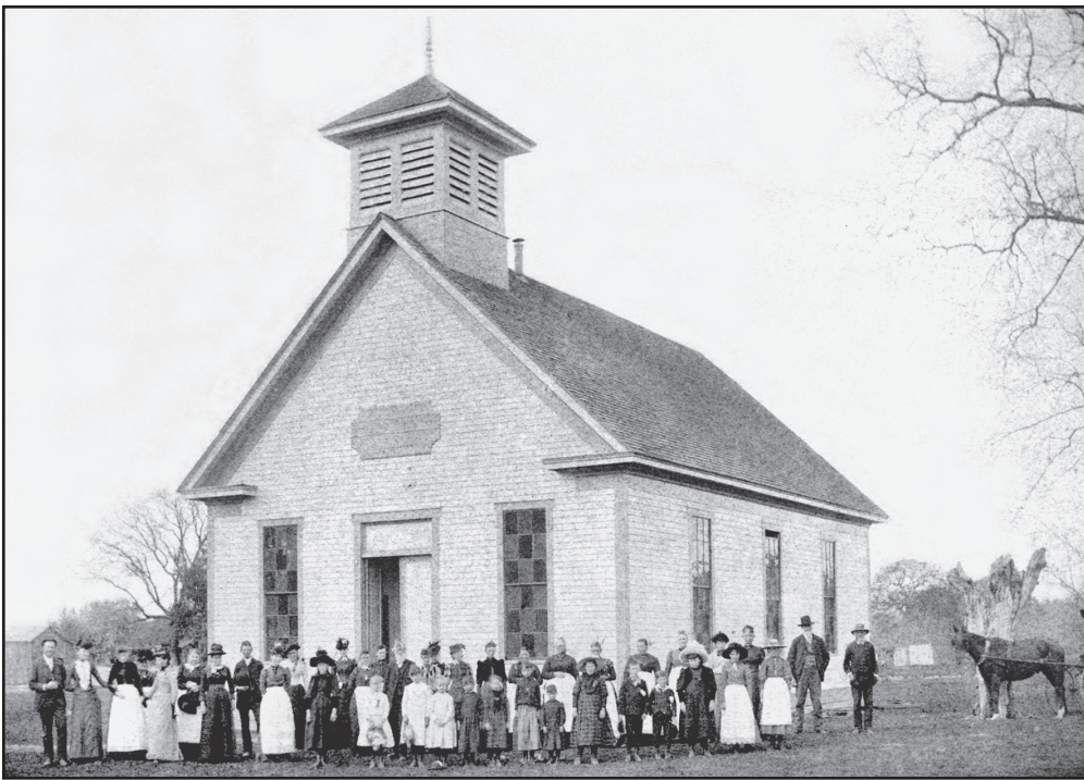
The Methodist Episcopal Church, built in East Windsor in 1863, photo ca. 1890.
