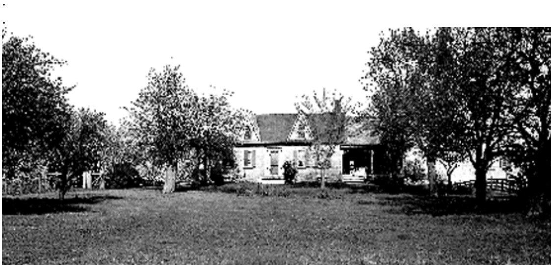
Home of Cyprian Winget where Esther Winget Warner's father was born 1857. A brick and stone porch was added before the MH Warner family moved here in 1915 (see page 46)
