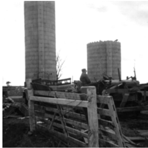
All that was left of the three silos
