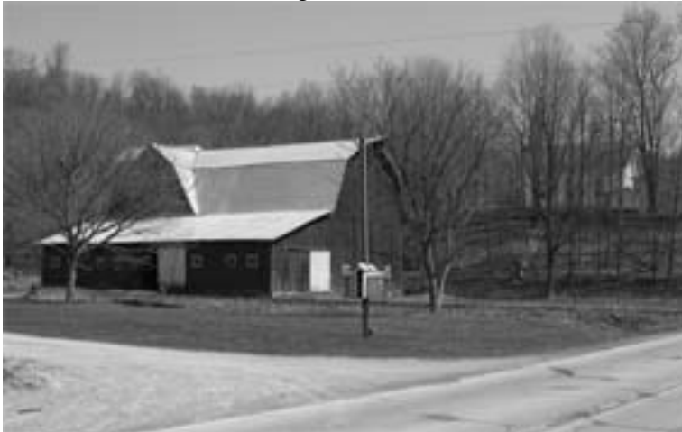
MH Warner barn built 1912
