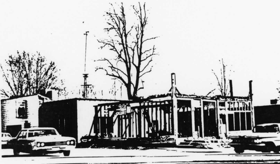
THE TEARING DOWN OF THE OLD OPERA HOUSE.
