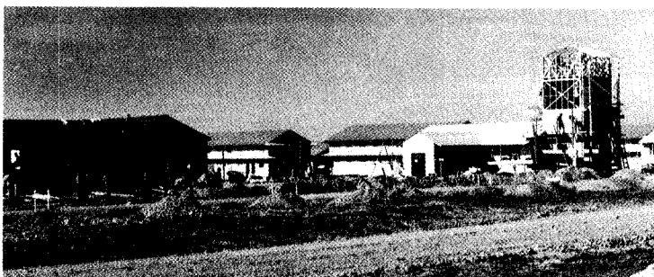
Construction at Pendleton
