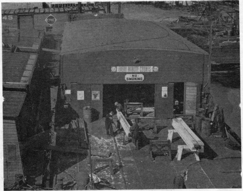
Temporary floating carpenter and blacksmith shop at Pier 2
