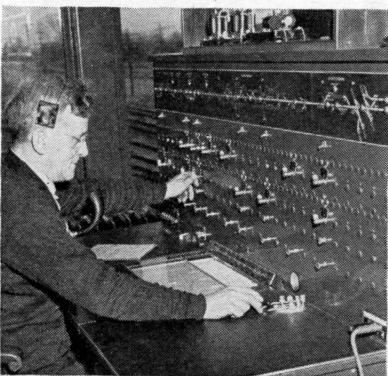
Operator C. J. Fenstermaker, in Leavittsburg tower, at the desk of the illuminated control board and penograph of centralized traffic control between Leavittsburg and Pymatuning
