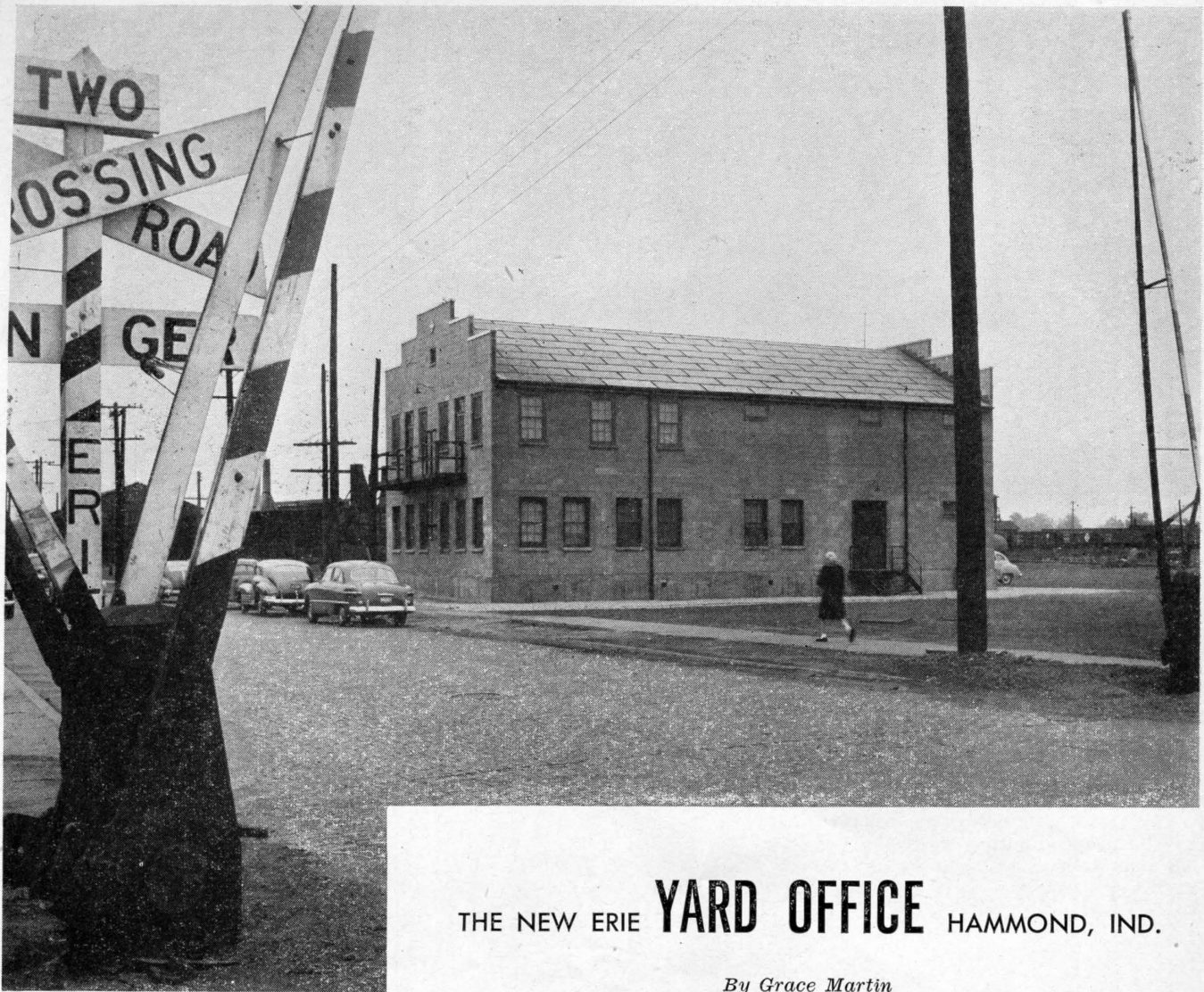
Looking across Douglas Street, from the east, at the new Hammond Consolidated yard office and rest rooms
