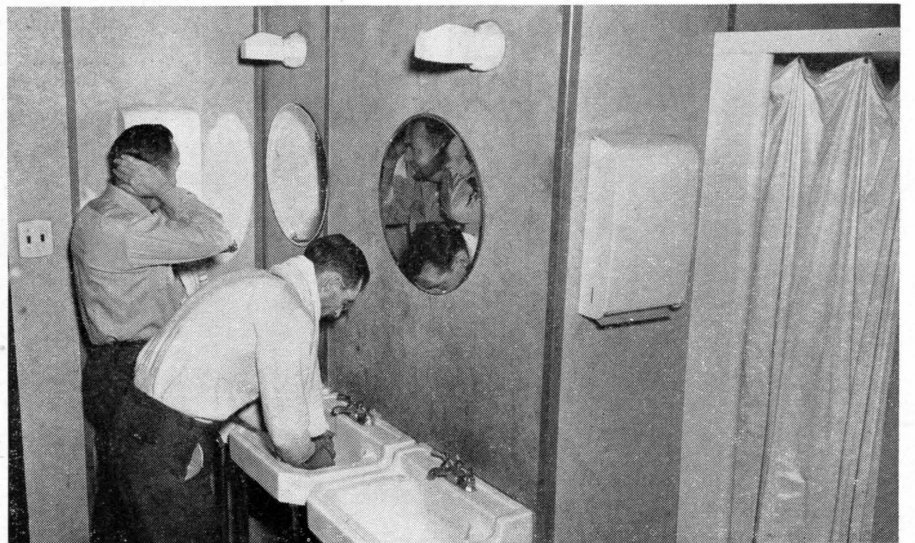
Brakeman I. G. Warkentien and Fireman F. E. Shockome in men's washroom on second floor. Showers and washbasins are a convenience to men in off the road. There are three enameled wash basins and also two shower bath stalls
