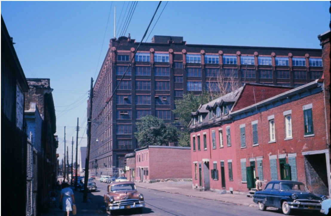
003QC - NE Shearer St. Building.
