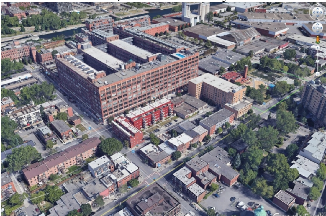
005QC - NE Shearer St. Building 2021
