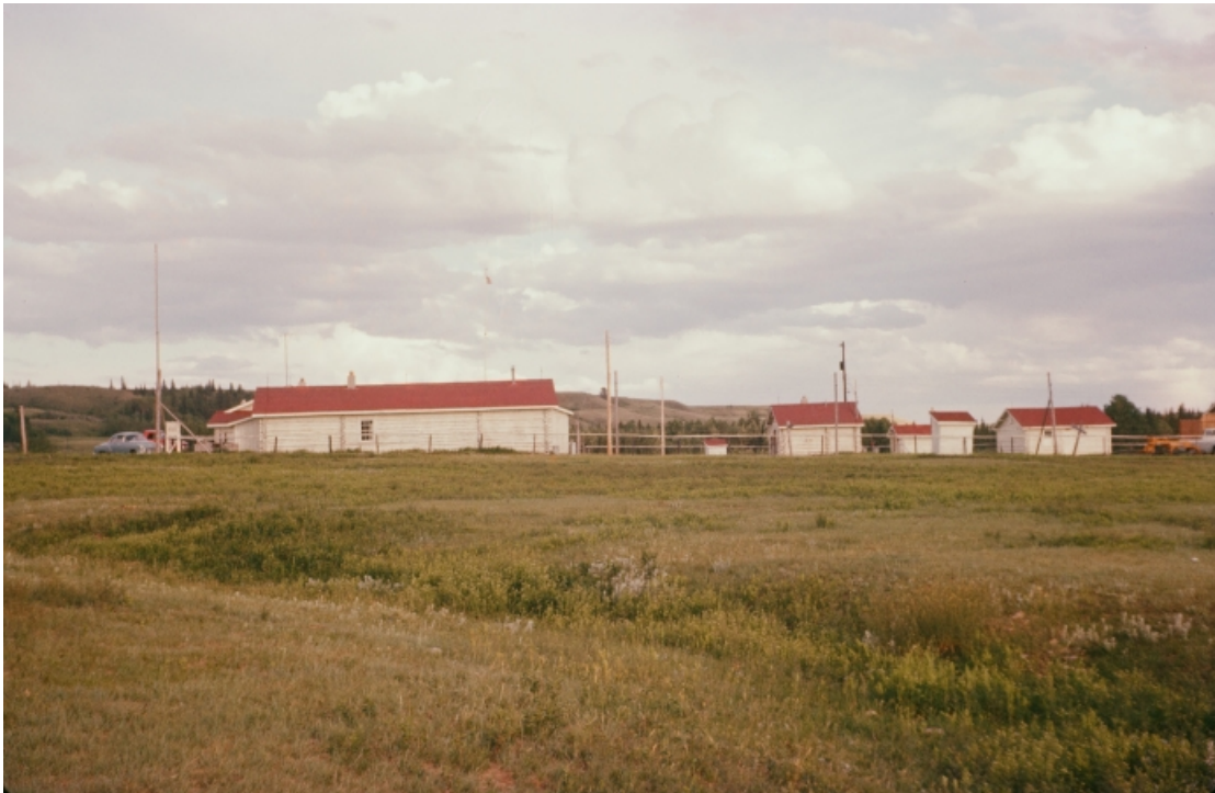
032SK - Fort Walsh Buildings. While we were doing the Survey in the West Block of the Cypress Hills, our meals were provided by the people at Fort Walsh. Very good home cooked meals. A bit of a break from restaurant meals at the restaurant at CHIP.
