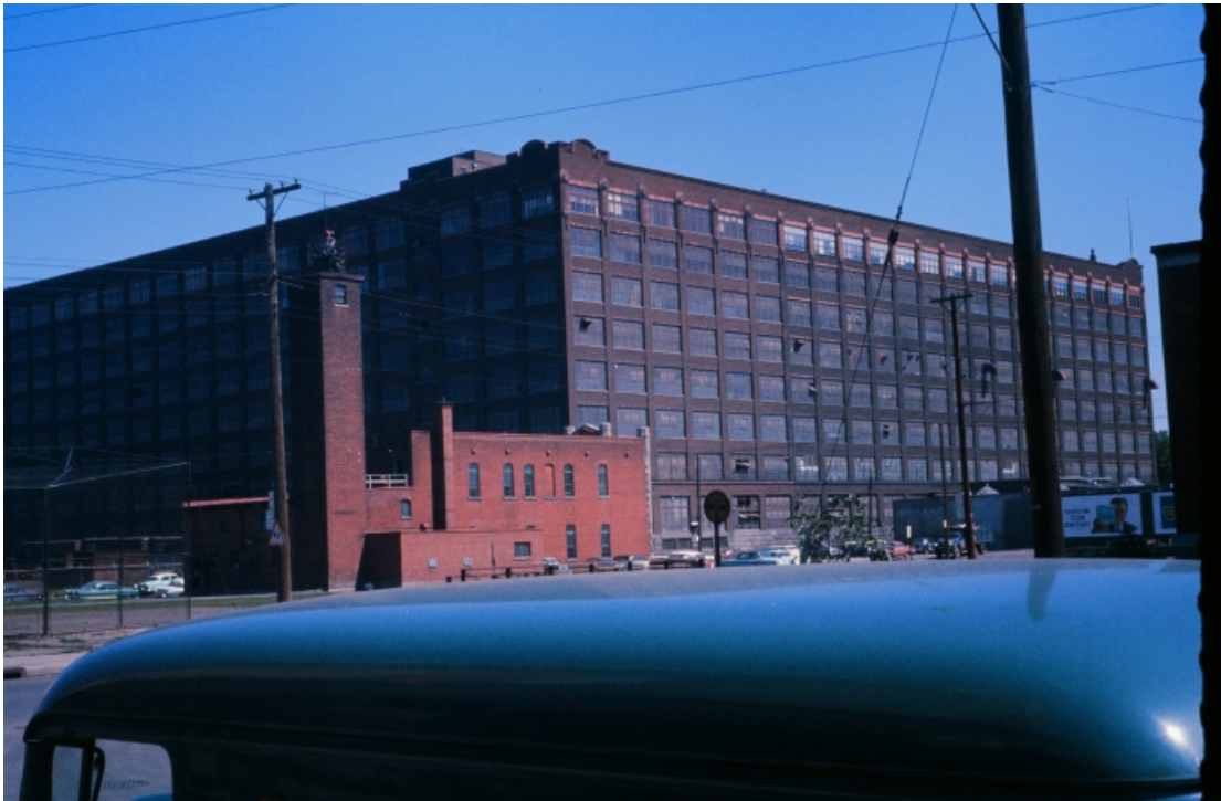
004QC - NE Shearer St. Building
