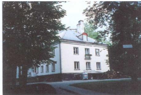
Manor in former Gramenz, Kreis Neustettin, Pommern, Germany
