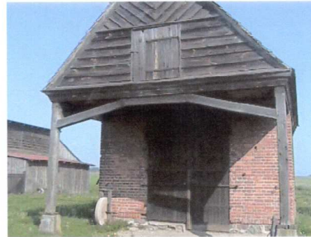
Blacksmith Shop in former Kreis Schlochau, West Prussia, Germany
