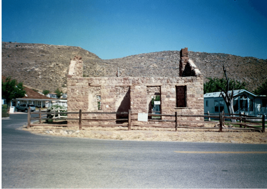
This home is located at the entrance to the RV Park
