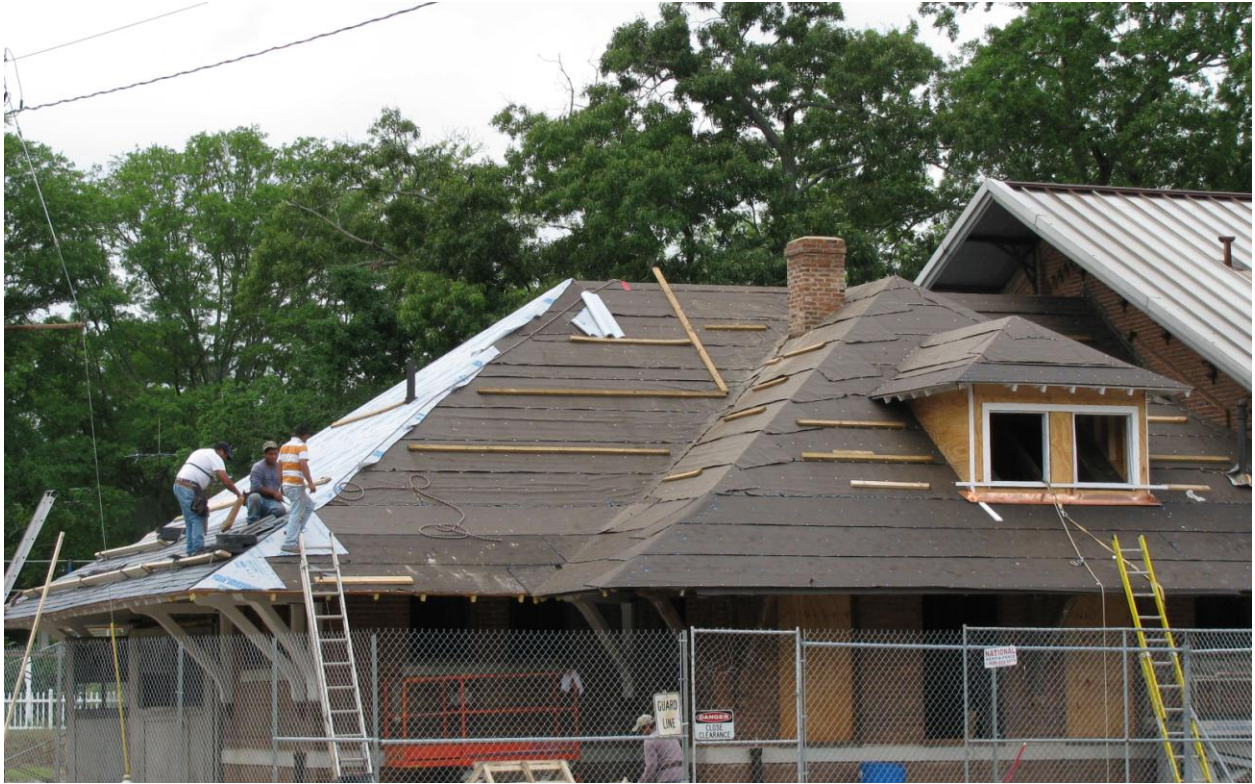
Here workmen are shown putting a slate roof on the waiting room section of the Depot. Below are more pictures of the new slate roofing.
