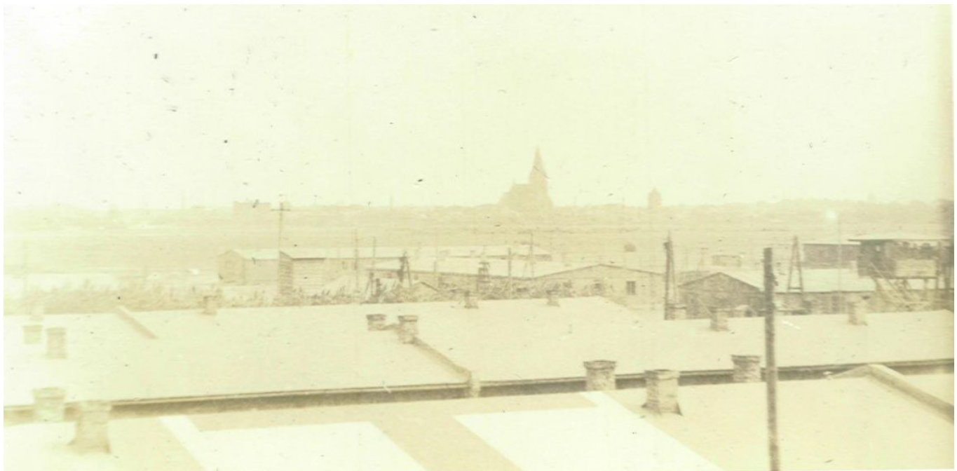
View towards Barth from tower shown in upper photo Note the prominent cathedral within the surrounding city wall front: camp hospital roof
