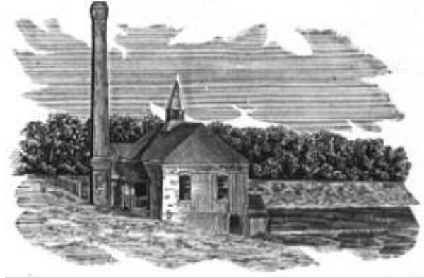
The Palatka Water-Works. The Pumping Station.
